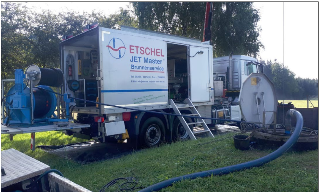
Figure 1: HPI-rehabilitation in Aichhalden
