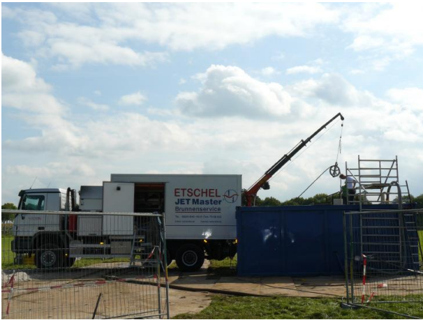
Fig. 13: The Johnson filter DN 300 is treated with JET Master
