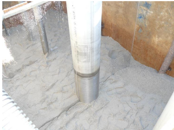
Fig. 12: Johnson filter screen is coated with sand
