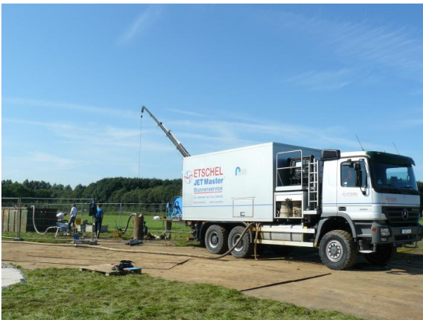
Fig. 6: well development with JET Master
