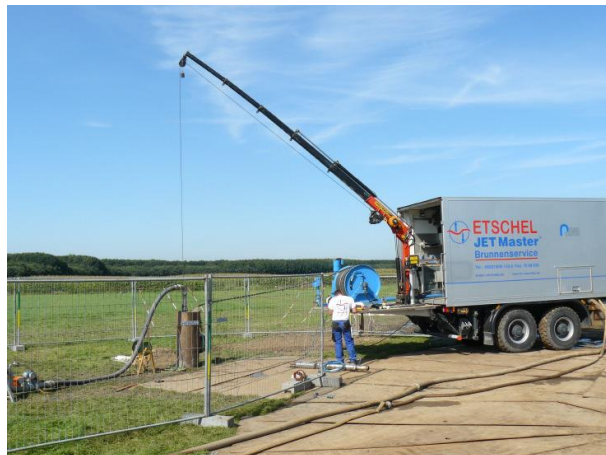
Fig. 7: HPI-Process with high water pressure and simultaneous pumping
