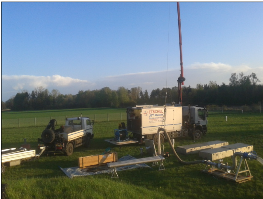
Figure 3: rehabilitation with the High Pressure Impulse-Process® with high water pressure, system JET Master®
